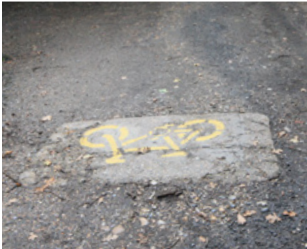
Existing signage, concrete pads in the path, protrude causing a hazard and are neither consistent nor clear.
